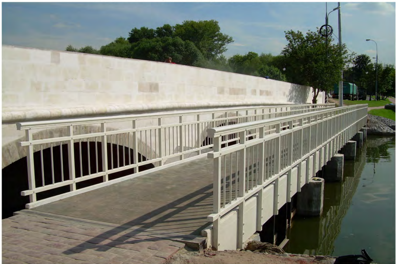
Pedestrian bridge on the Highway "Starokashirskoe"
