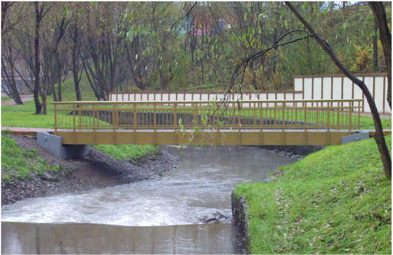
Pedestrian bridge across the river Lihoborka. Second construction stage. (bridge 1)
