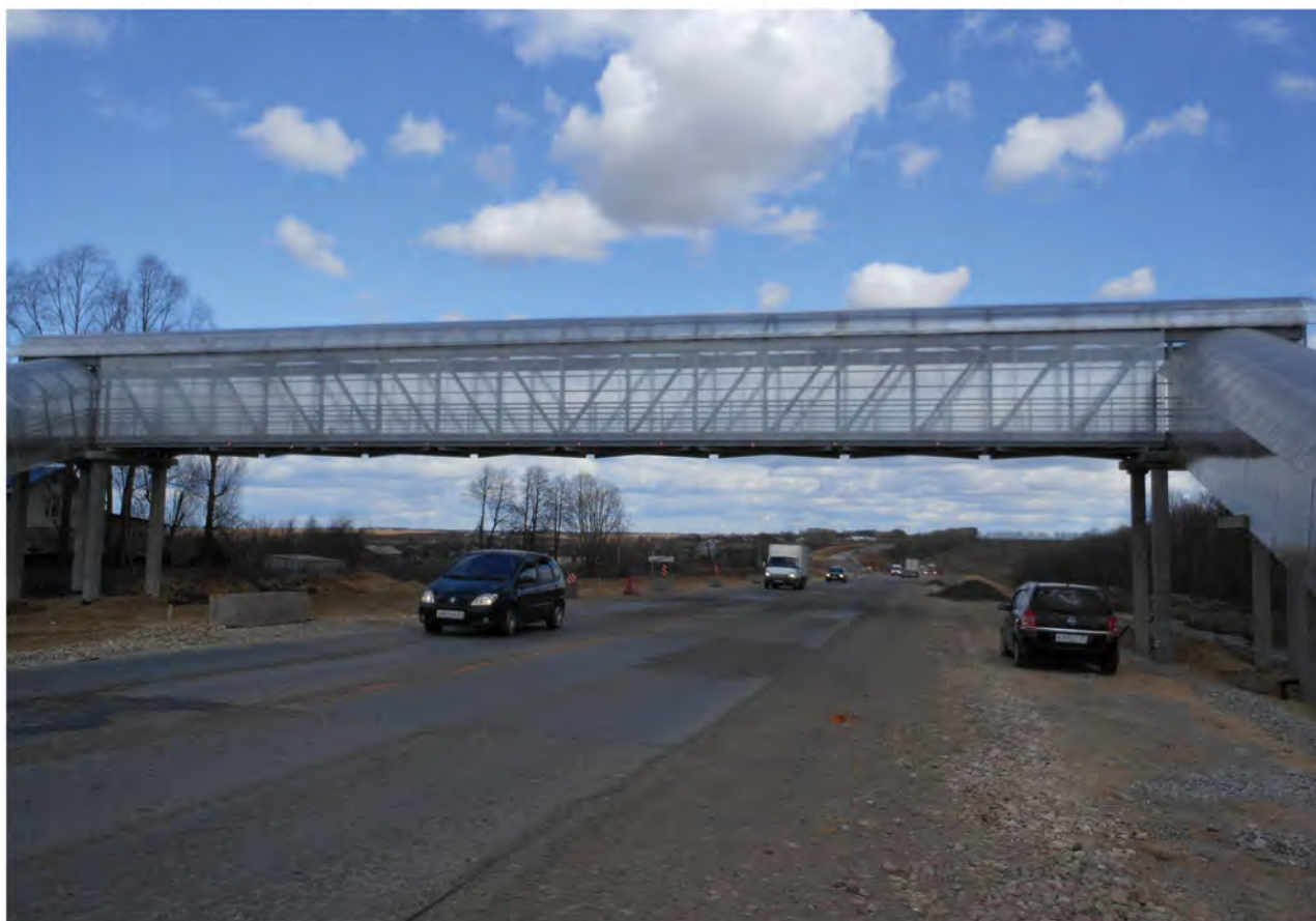
Bridge pedestrian crossing at 613+00 km - 623+500 km of the M7 highway
