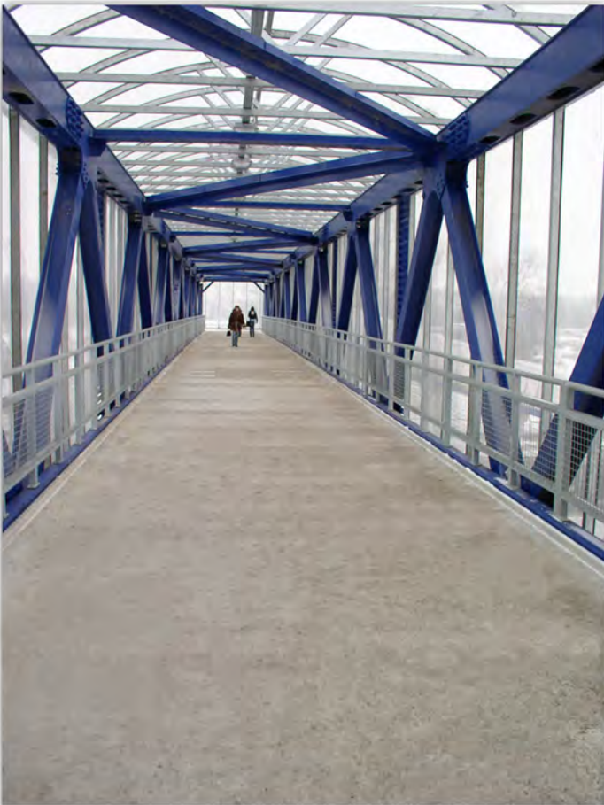
Composite plates-modules are transported from workshops of the enterprise and mounted in installation site.
