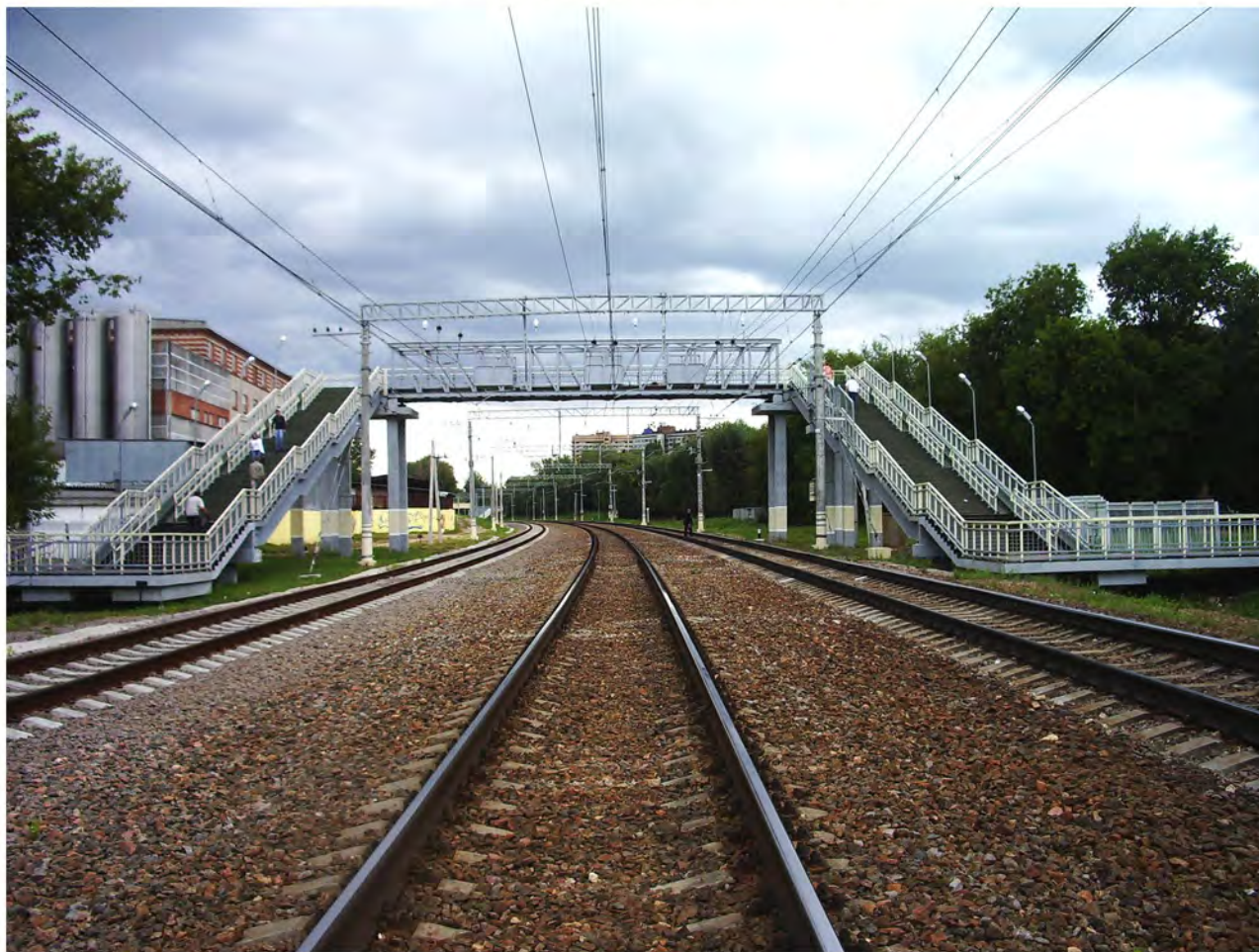
Pedestrian bridge Moscow-Kuskovo 7km.
