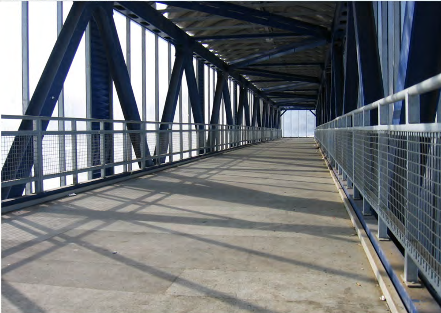
Air pedestrian crossing on 23rd km of Leningradskoe highway with deck made of ApATeCh composite materials
