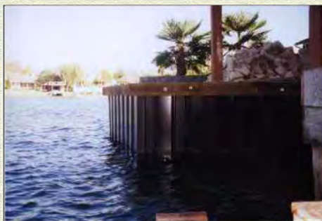
Step 8: The sheet piling is installed. The guaranteed service life is 70 years
