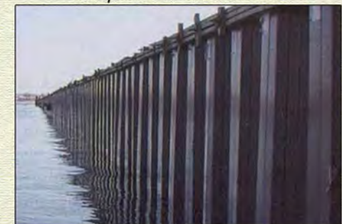
Step 8: The sheet piling is installed. The guaranteed service life is 70 years
