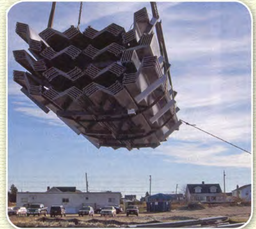
Profiles unloading on the site. Light weight of the profiles allows to unload by large consignments
