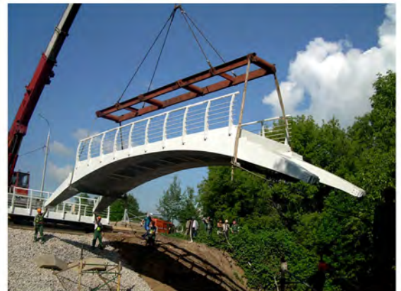
Stages of assembly on the site of arched bridge.
