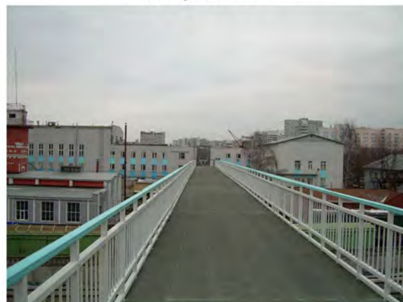
A new pedestrian passage with decking coating
