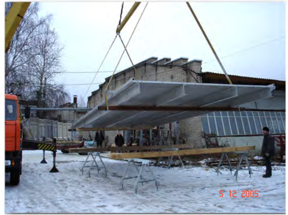
Composite plates-modules are transported from workshops of the enterprise and mounted in installation site.
