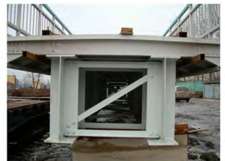
Assembling of the span on primary beam
