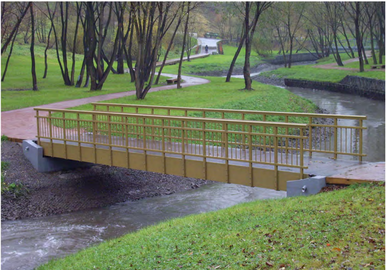
Pedestrian bridge across the river Lihoborka. Second construction stage. (bridge 2)
