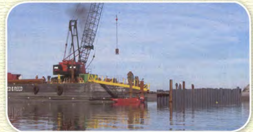
6-meter profile is stricken into the ground by using vibro-machine
