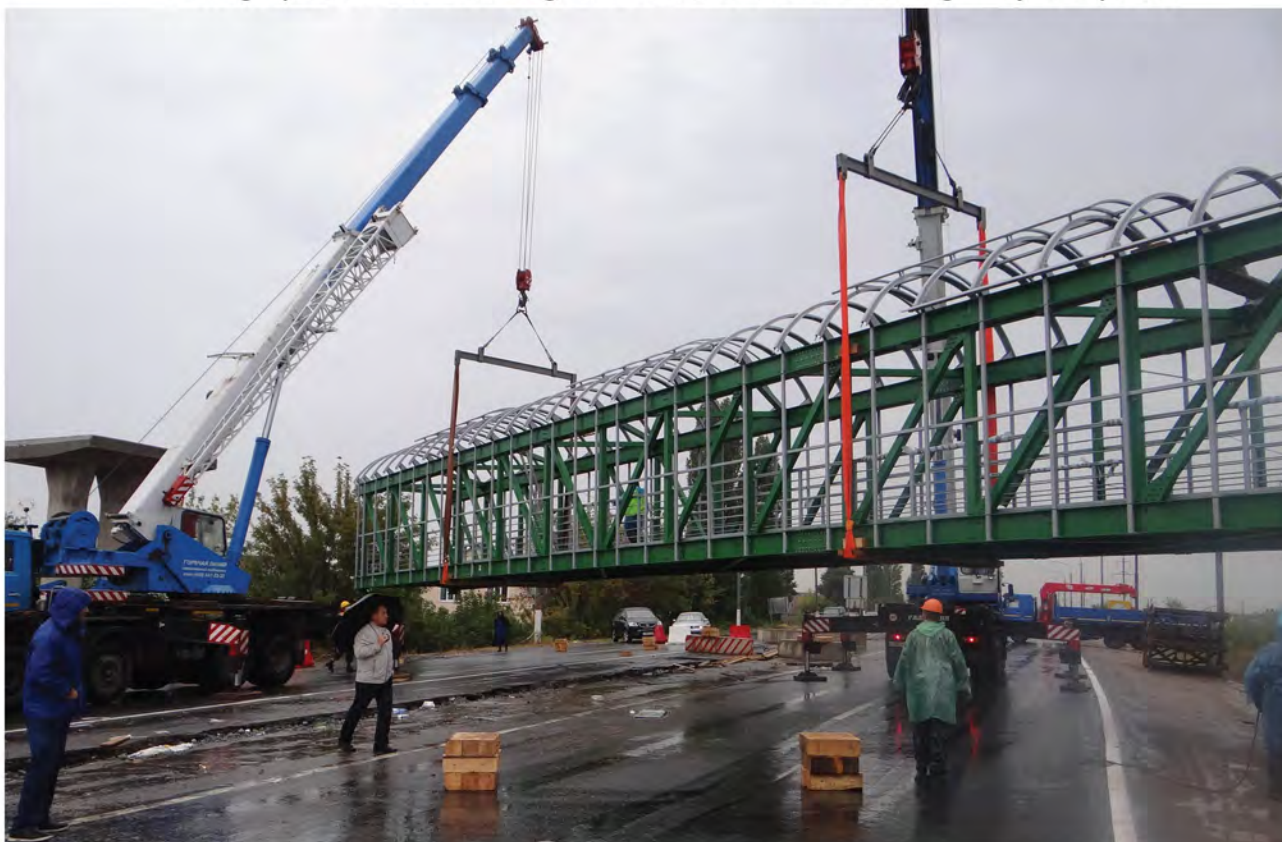
Bridge pedestrian crossing at 302 km of the 1P 119 highway in Lipetsk
