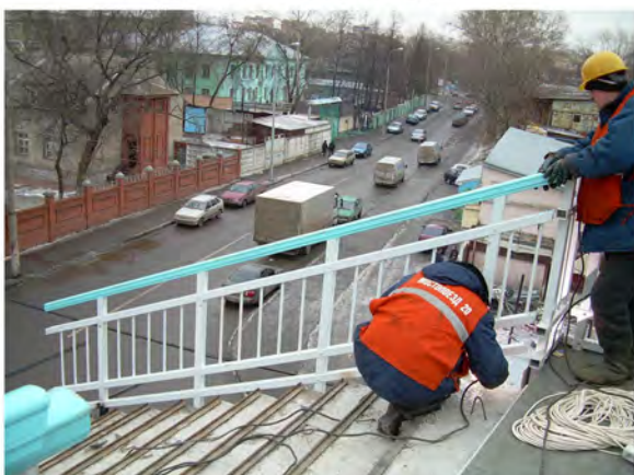
Installation of composite railings on reinforced-concrete stairs
